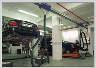
The Eurovac system can also be used with hose drops. A complete line of exhaust accessories are available.
