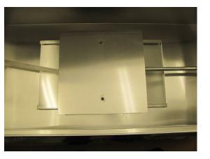
DAMPER options includebutterflytype,LowPressureDrop(LPD)damperandguillotinedamper(seeabove,guillotinedamperisabove the diffuser plate).
