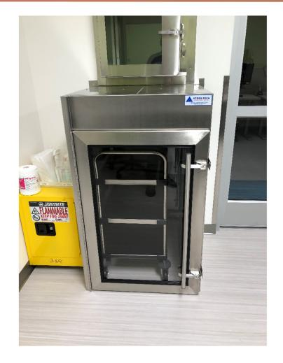
Available Options include: HEPA/ULPA Filtration & Fan Standard & Ultra-violet Lighting Automatic And Vertical Sliding Doors Fire Rated Doors
