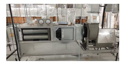
**Filter-Fan Units** can be packaged with any in-line filter housing. HEPA/ULPA filter housings can be mated to utility fans and they can also be put into series with other filter housings including carbon-tray or carbon-canister housings to address both chemical/odor and particulate capture. *(see pic at left of HEGA-HEPA filter fan unit)*
