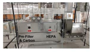
Mounted, and can provide pressure-drops transmitted to Bldg. Automation Systems
