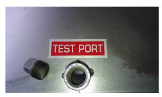
**DOP Test Ports** are available for HEPA/ULPA filter challenge. (see pic at left)
