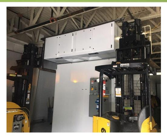
For large, custom showers like the one pictured here, site assembly by an experienced installer is mandatory. This model AS8109 (8'x10'x9' ID) shower with two high-speed roll-up doors arrived at the site in (3) large crates, weighing approx. 5000-lbs. Installing the two top-mounted filter-fan cabinets required a lot of finesse, given only a few inches of clearance to the trusses above.
