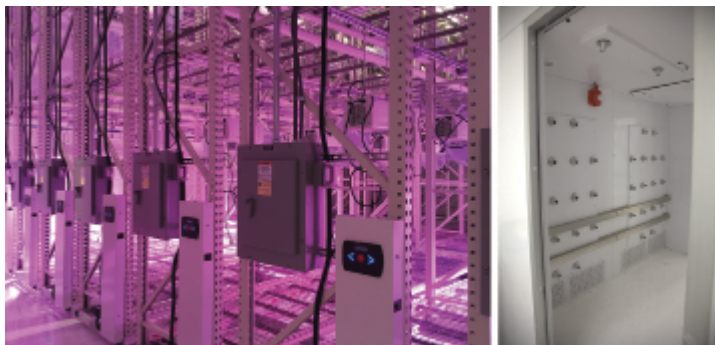
Left: American Cannabis Company’s HDCS (High Density Cultivation System), which takes advantage of vertical space while utilizing the maximum square footage possible. Right: An air shower can be effective for entry into clean zones. Photo courtesy of American Cannabis Company
