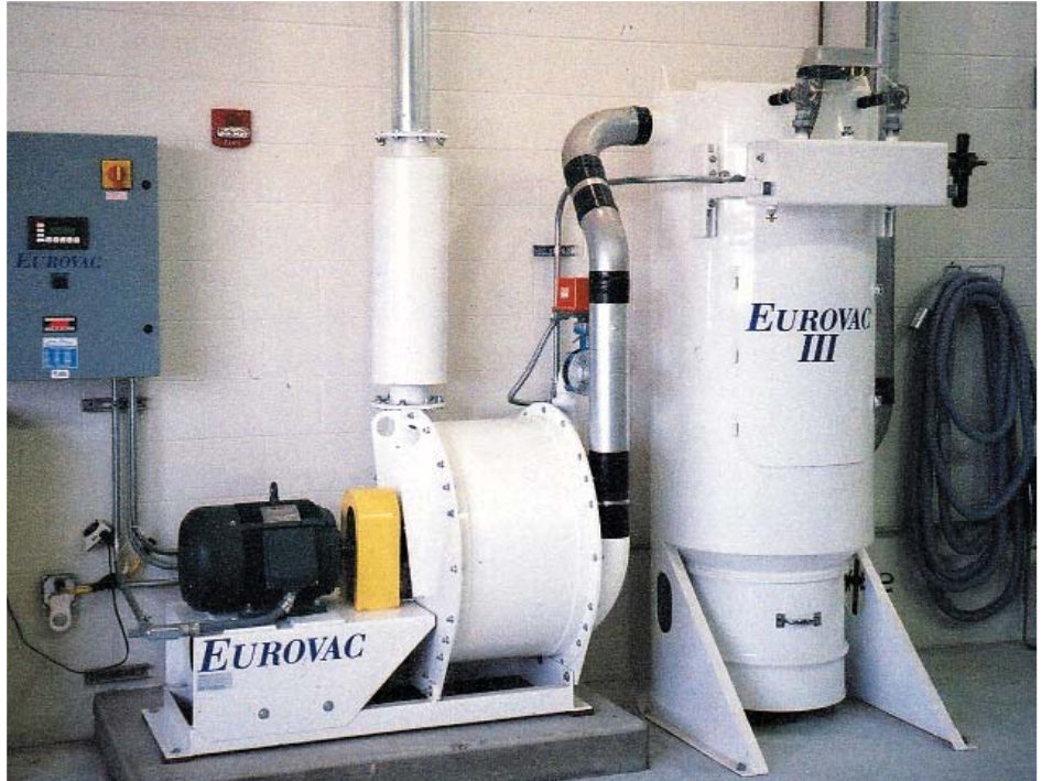
Eurovac III System with 20HP Centrifugal Multi-Stage Pump and 30" Separator
